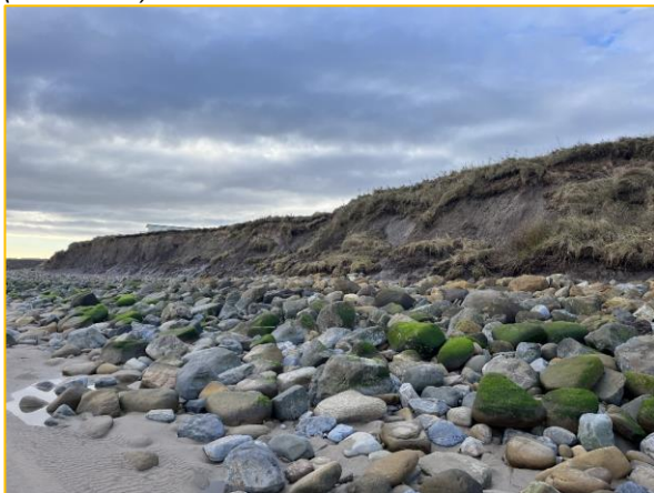
Actively eroding cliff between breakwaters and River Wansbeck (/3701C03)
