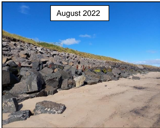
New rock armour placed at toe to create a stable slope, protecting the damaged steel (/4001C02)
