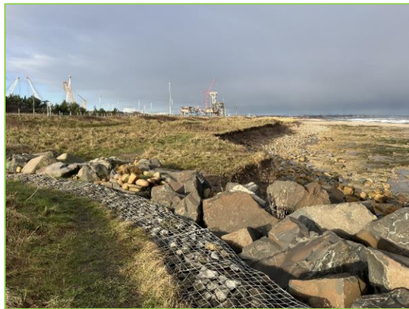
Rock revetment buried northern tie in (/4001C01)
