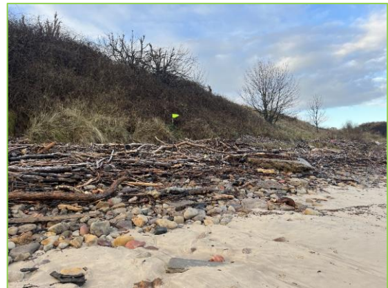
Lower beach levels and storm deposits at the toe of the cliffs (/3801C02).
