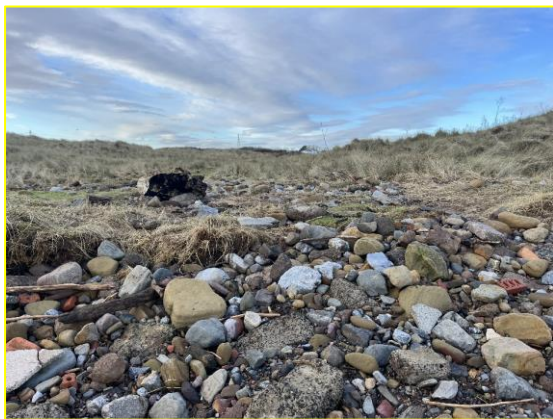
Overtopping evident during recent storms (/3801C01)
