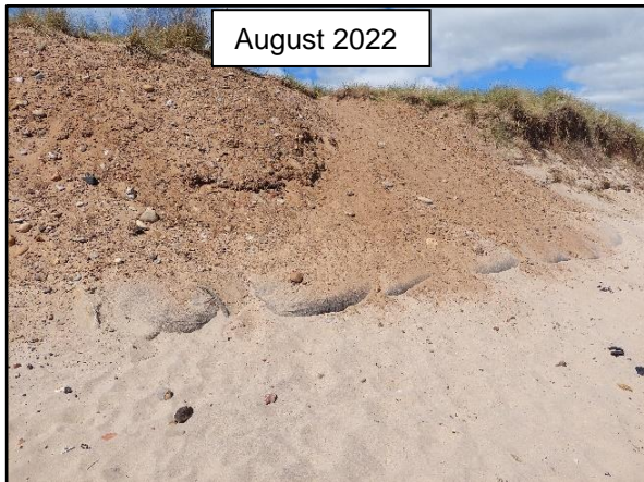
Sandbags and reinstated dunes at cable landfall layout (/3901C04)
