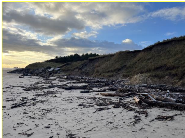
Waterline cut back with moderate toe erosion (/3901C01)
